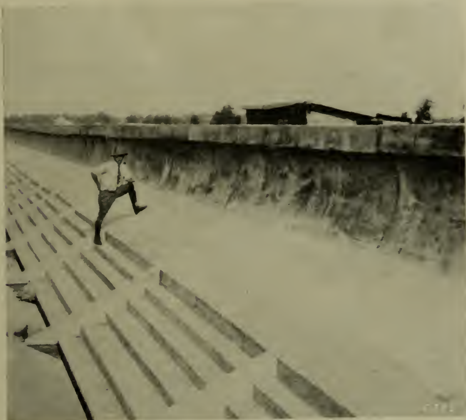
FIG. 7. NEW SEA WALL. EAST COAST.
